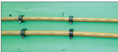
Figure 3.3.1 Installed piping services prior to the installation of Hebel PowerPanel 50
